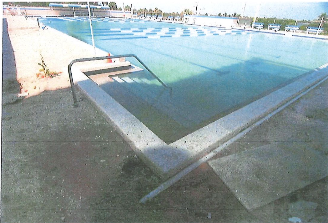
EXHIBIT 6. VIEW OF STEPS IN NORTHEAST AREA OF POOL
